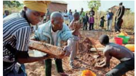
Villagers making adobe bricks to build a new childhood center in Ng'andu, Malawi.
